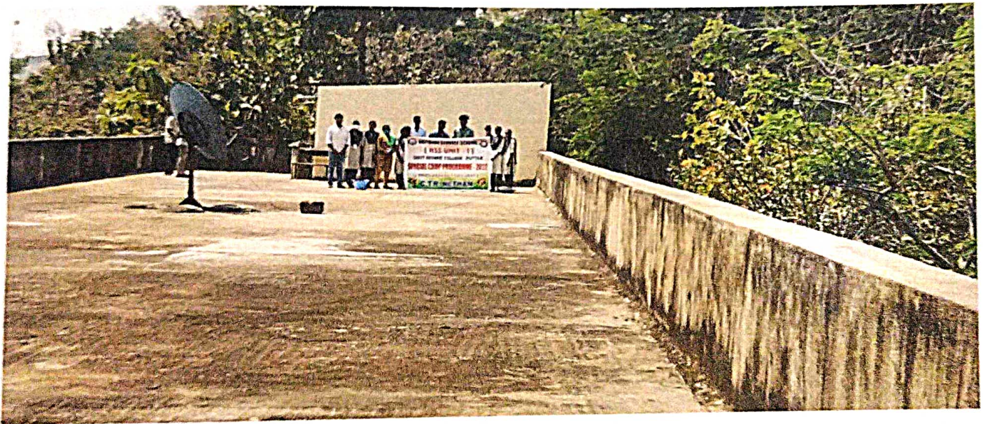
Seminar Hall Terrace Cleaning
